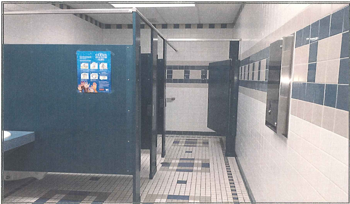
BATHROOM FINISH IN GYMNASIUM BUILDING
